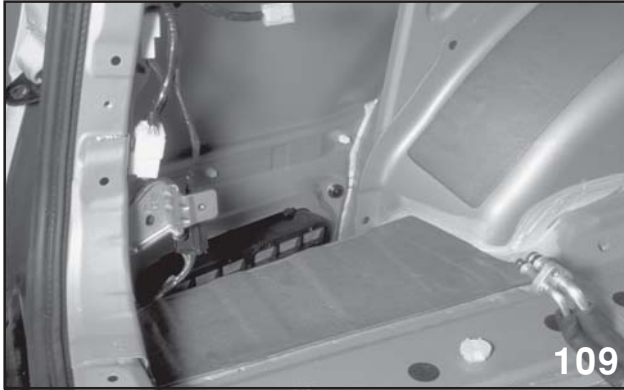
Rear Evaporator Removed
